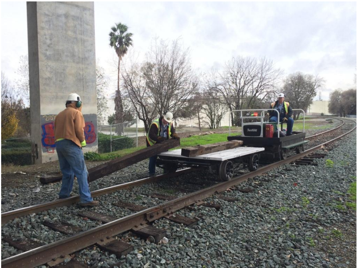
Steve and Frank load dead ties onto the flat car which Chris will shuttle down to the Setzer yard
