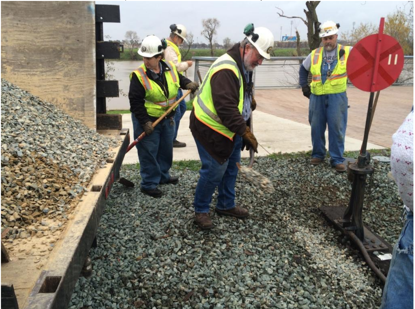
Frank and Heather shovel small rock around the head-block at Switch 11 – North Clunie
